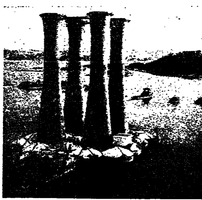
A symbol of Norway's new wealth: the base of Statfjord C being towed to a deep water site
